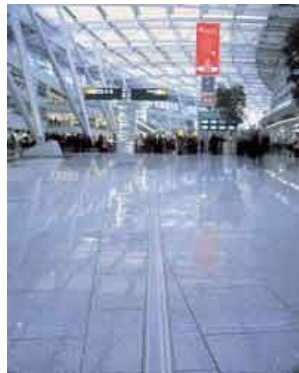
FS 110 virtually disappears in granite airport floor. (Click image to enlarge)
