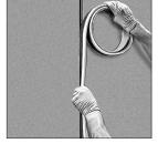
Work your way along the joint pinching the material while inserting it.
