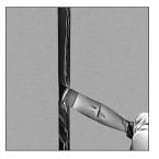
Strike the mounting bead of liquid sealant with a caulk knife to ensure that it is continuous, even, and encapsulates the old sealant residue.
