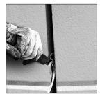
Remove old sealant using a long-bladed utility knife. This can be accomplished in two cuts. The first to remove most of the sealant and backer-rod and the second to trim out remnants of old sealant. Take care to not damage the underlying substrates.
