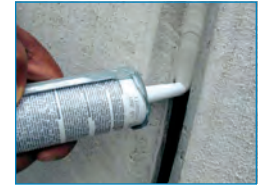
Backerseal behind field-applied liquid sealant provides true "belts and suspenders" sealing – 2 systems working on different principles to guarantee performance of the same function.
