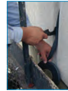
Backerseal behind field-applied liquid sealant provides true "belts and suspenders" sealing – 2 systems working on different principles to guarantee performance of the same function.
