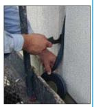
Insert the lengths to be joined into the joint-opening in the wall. Always push the material toward the join to prevent stretching. DO NOT PULL—this will cause the joins to separate after the stretched material shortens over time and will result in a gap where leaks could occur.
