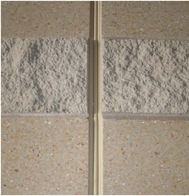
A fire-rated expansion joint set in place which maintains the performance properties of the interior wall system. The watertight silicone outer seal of the precompressed, impregnated foam joint is manufactured to color coordinate with the tile and stone façade of the wall. - EMSEAL Photo
