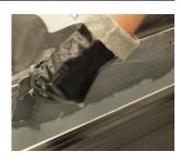
IMPORTANT: While one or more workers are applying epoxy to the joint faces, others must prepare the SJS-FP foam/spline assemblies.
