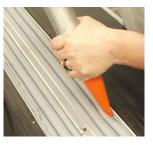
IMPORTANT: On installations of long runs of material, have one worker drop back after the installation of the first several lengths to install the silicone sealant bands before the epoxy cures.
