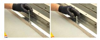
Remove excess epoxy from around the nut that might obstruct tightening later. Allow epoxy to cure according to chart(s) on epoxy cartridge.
