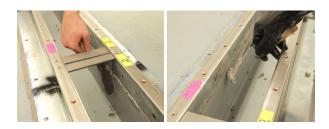
Tool epoxy along the outer edges of the mounting flanges into a cantstrip to make a ramp for the deck waterproofing material.
