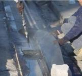
sheet. Release the FP flashing sheet and press it into the membrane — BE SURE to press the flashing sheet firmly into the corner between the leg and the mounting flange. Eliminate all bubbles and puckers.
