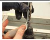
Drill 3/8" diameter holes for the 5/16" diameter anchors (or as otherwise specified for the particular job or anchoring system-- consult EMSEAL).
