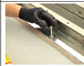
Remove excess epoxy from around the nut that might obstruct tightening later.
