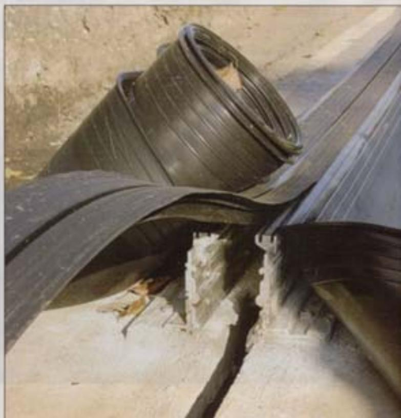
problem with this is that the accumulation of water combined with freeze/thaw cycles, flex fatigue from movement, and abrasion between topping and buried components results in the inevitable rupture of the buried "band-aid." Repair then involves removing the entire surrounding top-
