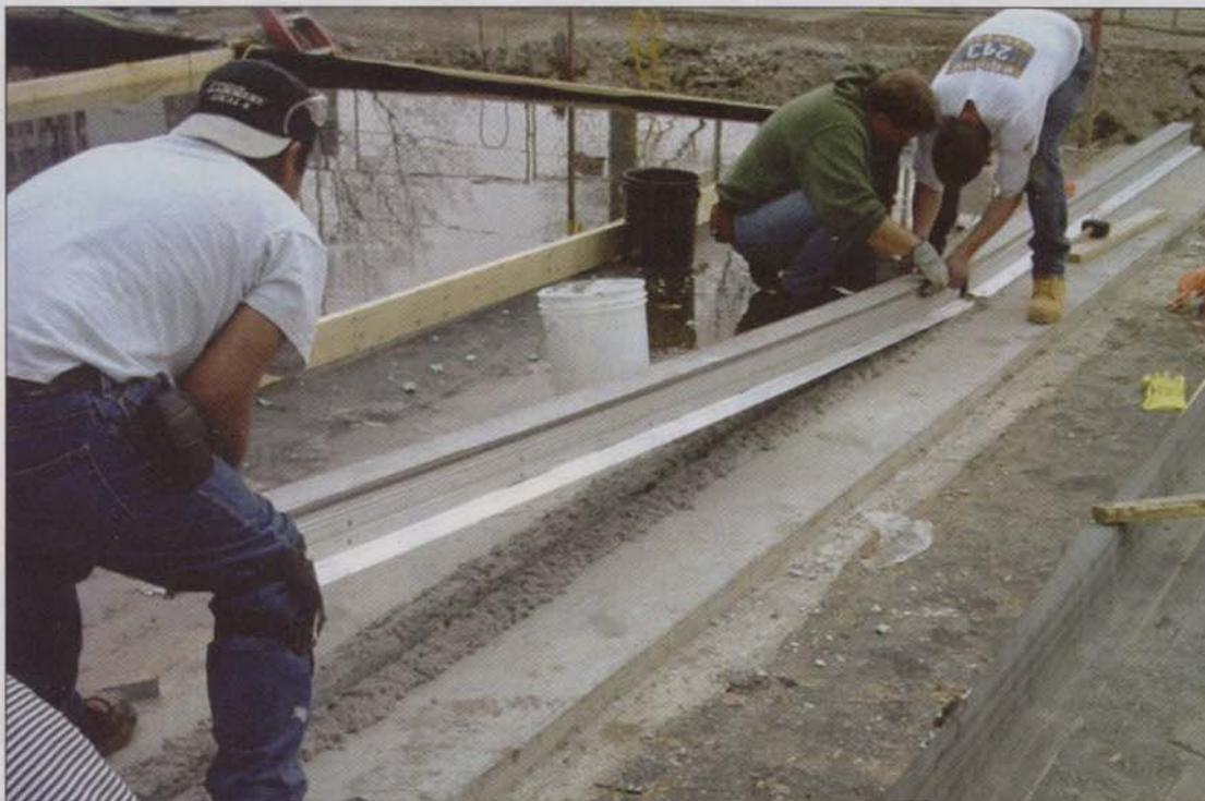
Mounting rails are lowered into position into an epoxy leveling bed.
