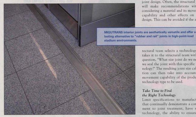
tectural team selects a technology and takes it to the structural team with the question, "What size joint do we need if we seal the joint with this specific technology?" The resulting joint size calculation can then take into account the movement capability of the product or technology type to be used.
