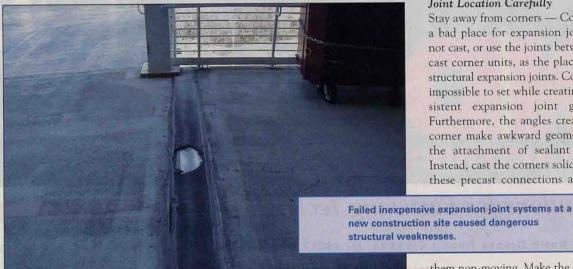
them non-moving. Make the structural expansion joint in a straight line just off the corners.
