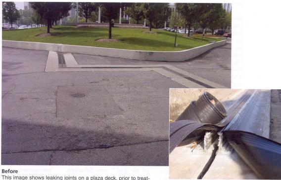
This image shows leaking joints on a plaza deck, prior to treatment with EMSEAL's MIGUTAN joint sealing technology.
