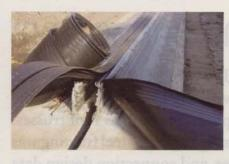
Migutan system components — retainer legs installed onto structural slab, side flashing sheets and movement gland - before installation of stainless steel retaining caps and before integration into the deck waterproofing membrane.
