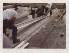
Mounting rails are lowered into position onto an epoxy leveling bed.
