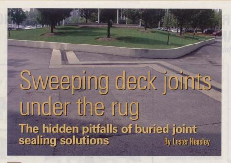
eck expansion joint sealing is critical to parking structure performance and longevity. Even more critical than watertightness of joints is parking deck design that incorporates a structural slab waterproofing membrane under a wear-course or topping slab. Until the emergence of a watertight, purposedesigned system, designers were left with the ineffective option of a buried looped membrane "band-aid" approach to address these critical joints.
