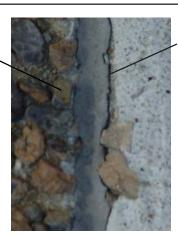
Liquid-applied sealants rely on adhesion. Adhesion is weakest in tension. As structures expand and contract with thermal changes, liquid-sealants eventually separate from substrates.
